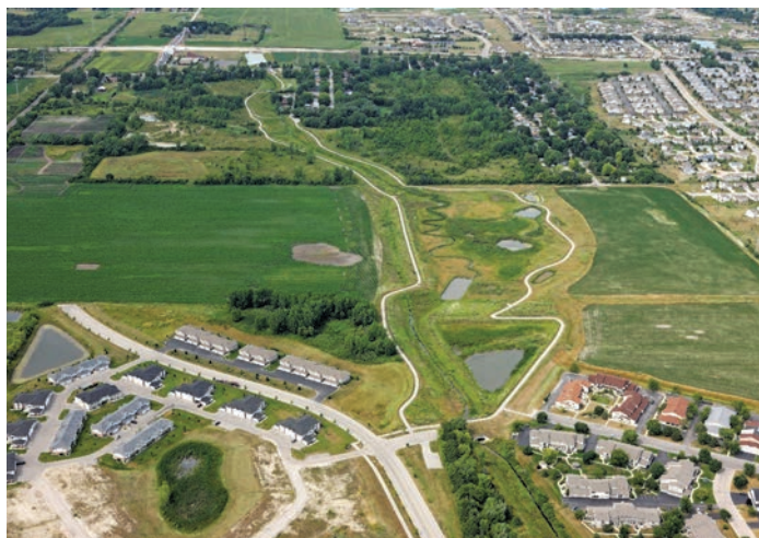
Phase 1 of the project. The recreational trail surrounds a large flood storage area containing a reconstructed meandering section of the river and various wetland/water quality features.
