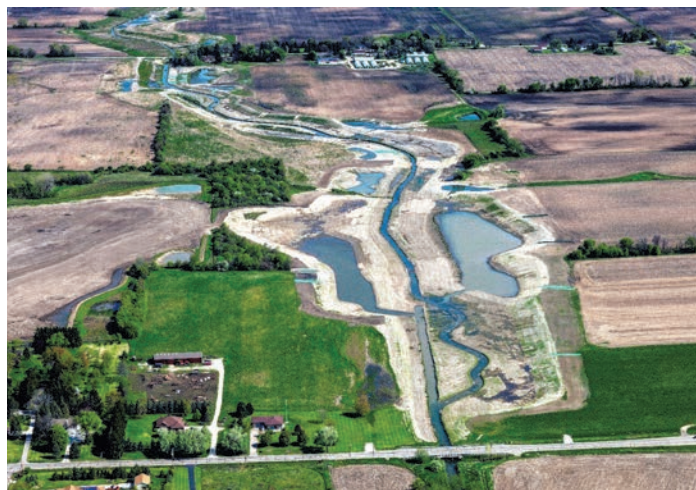
Phases 8 and 9 of the project shown under construction.
