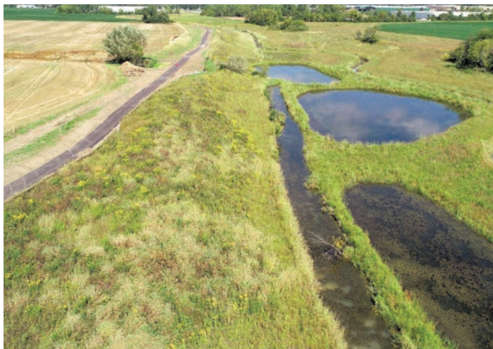
Phase 7 of the project. The recreational trail runs parallel to the newly constructed stream and ponds.
