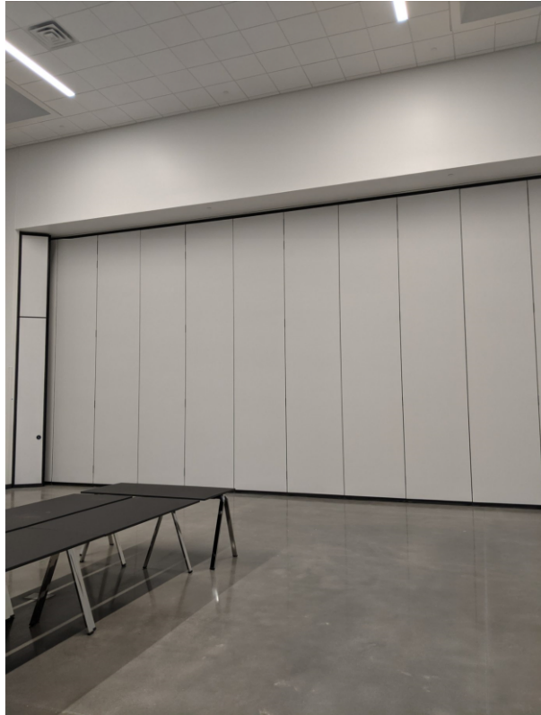
Install operable partition in cafeteria/lounge area
