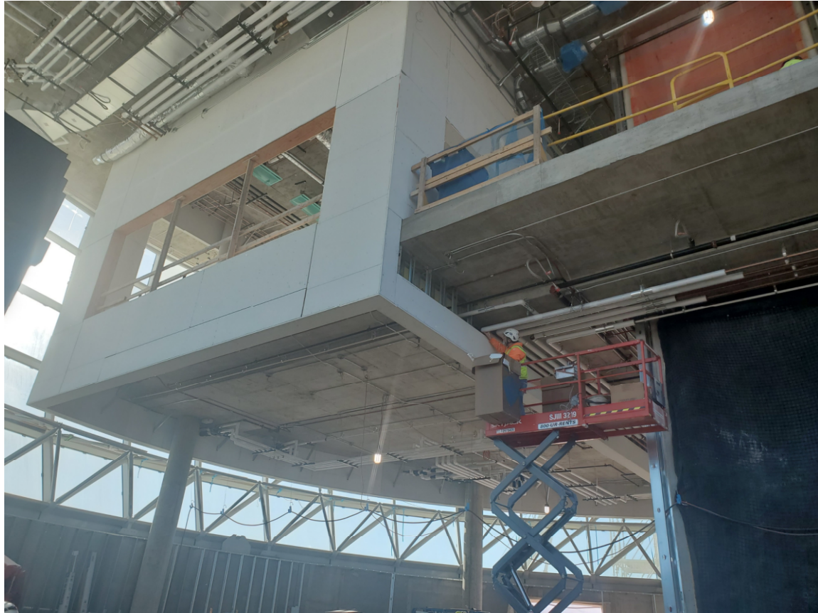
NOC Wall Framing
