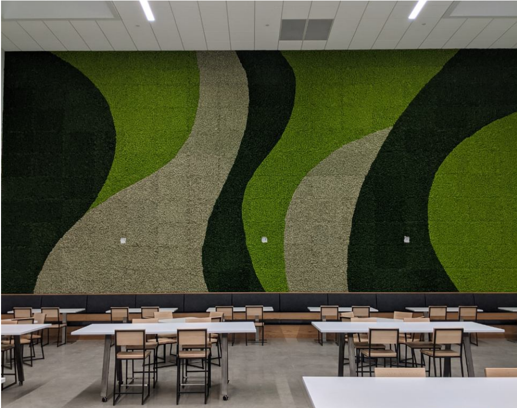
Complete installation of moss wall in the cafeteria/lounge area
