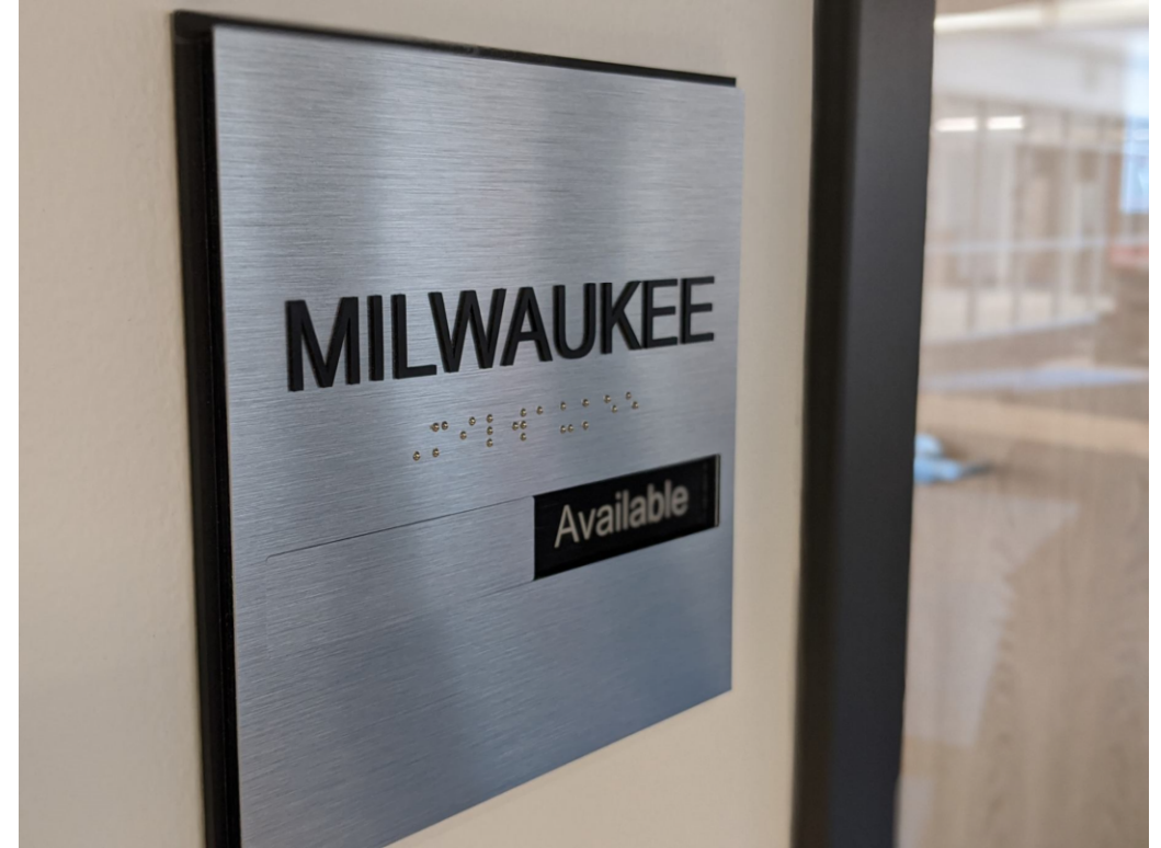
Install interior signage throughout the building
