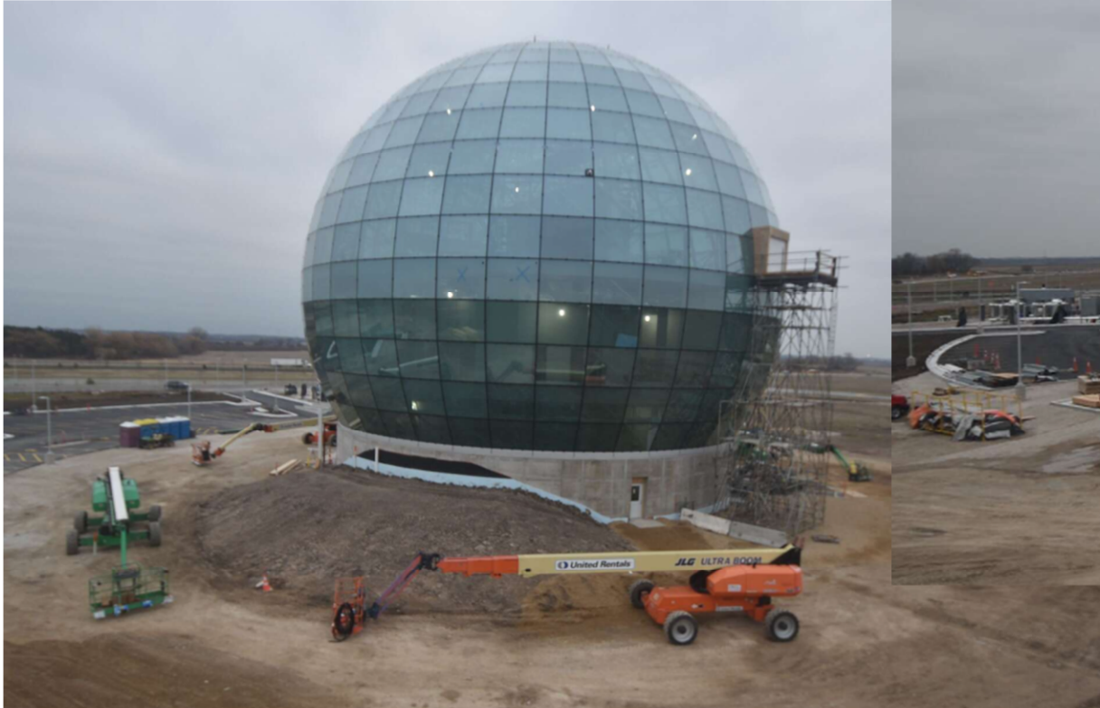
Data Center Structure – West View
