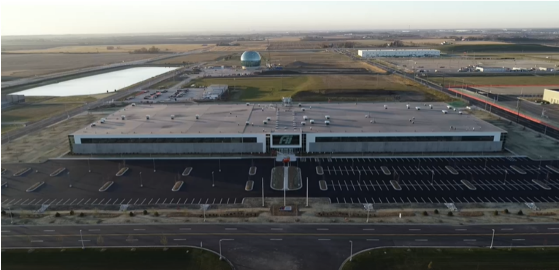
Complete striping of north parking lot
