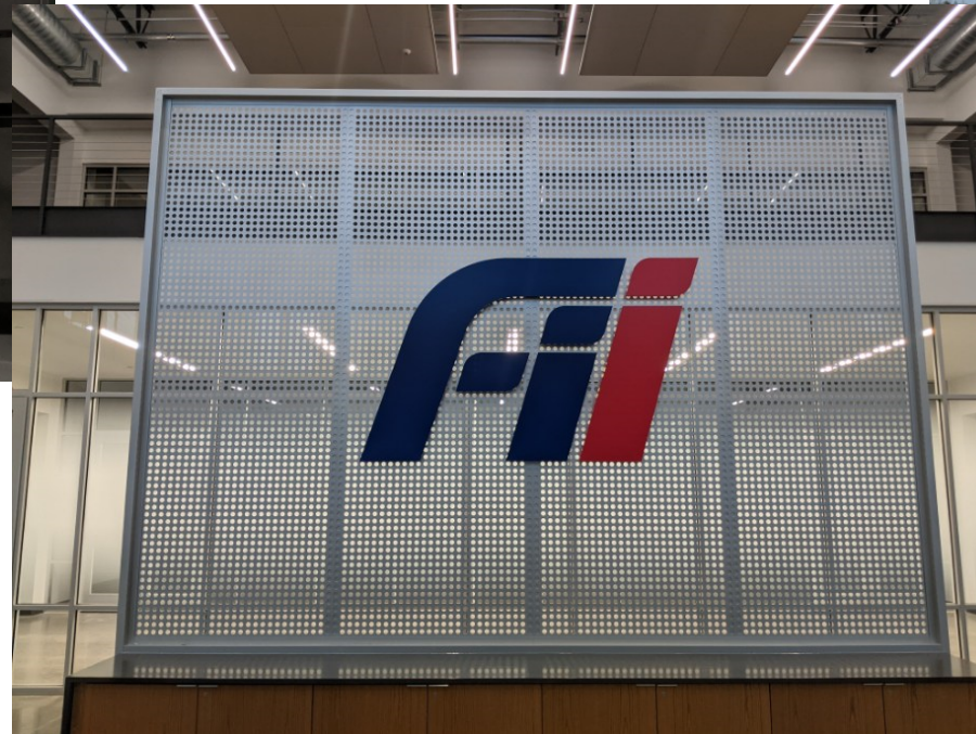
Reception sign installation begins in vestibule
