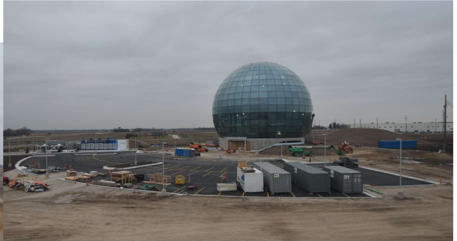
Data Center Structure – North view
