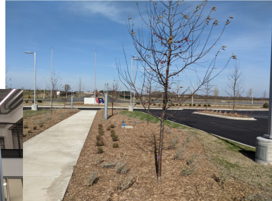
Complete exterior landscaping at the front parking lot
