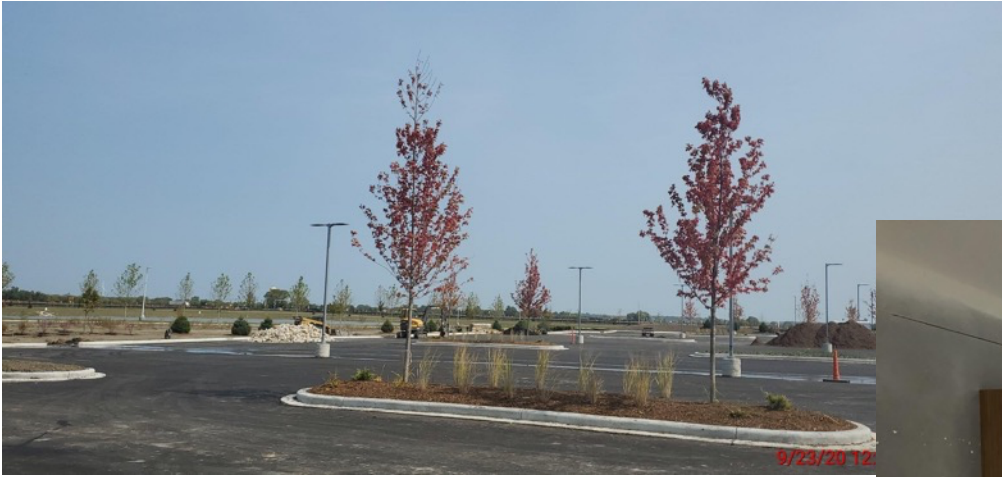
Begin landscaping in the north parking lot
