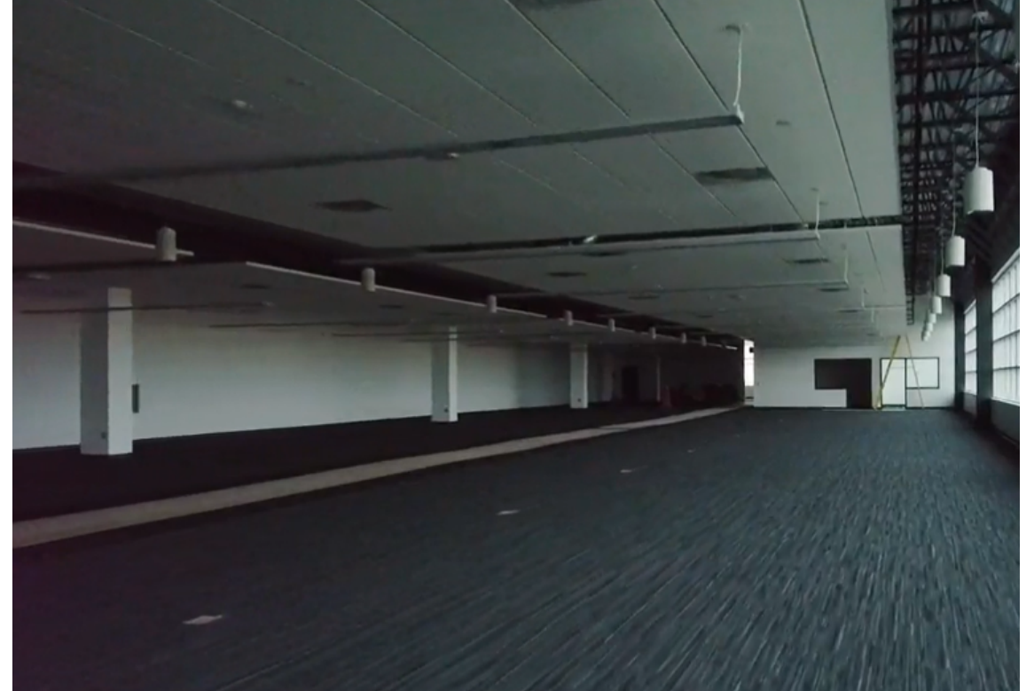
Completing carpeting and lighting on the mezzanine
