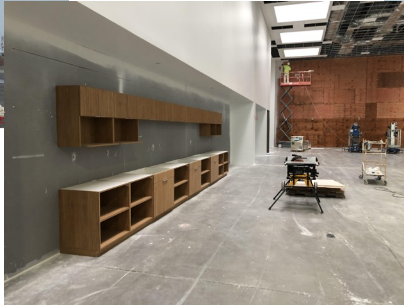
Begin installation of the casework in the cafeteria/lounge area
