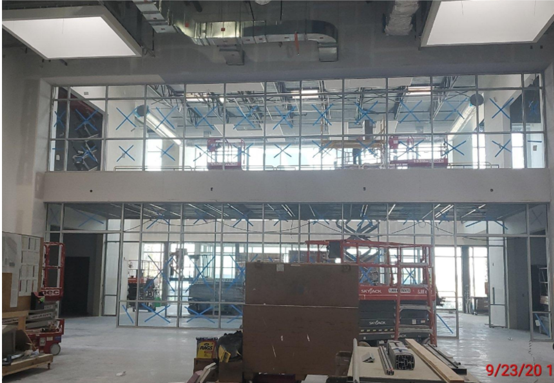
Installation of the aluminum storefront on the mezzanine bridge
