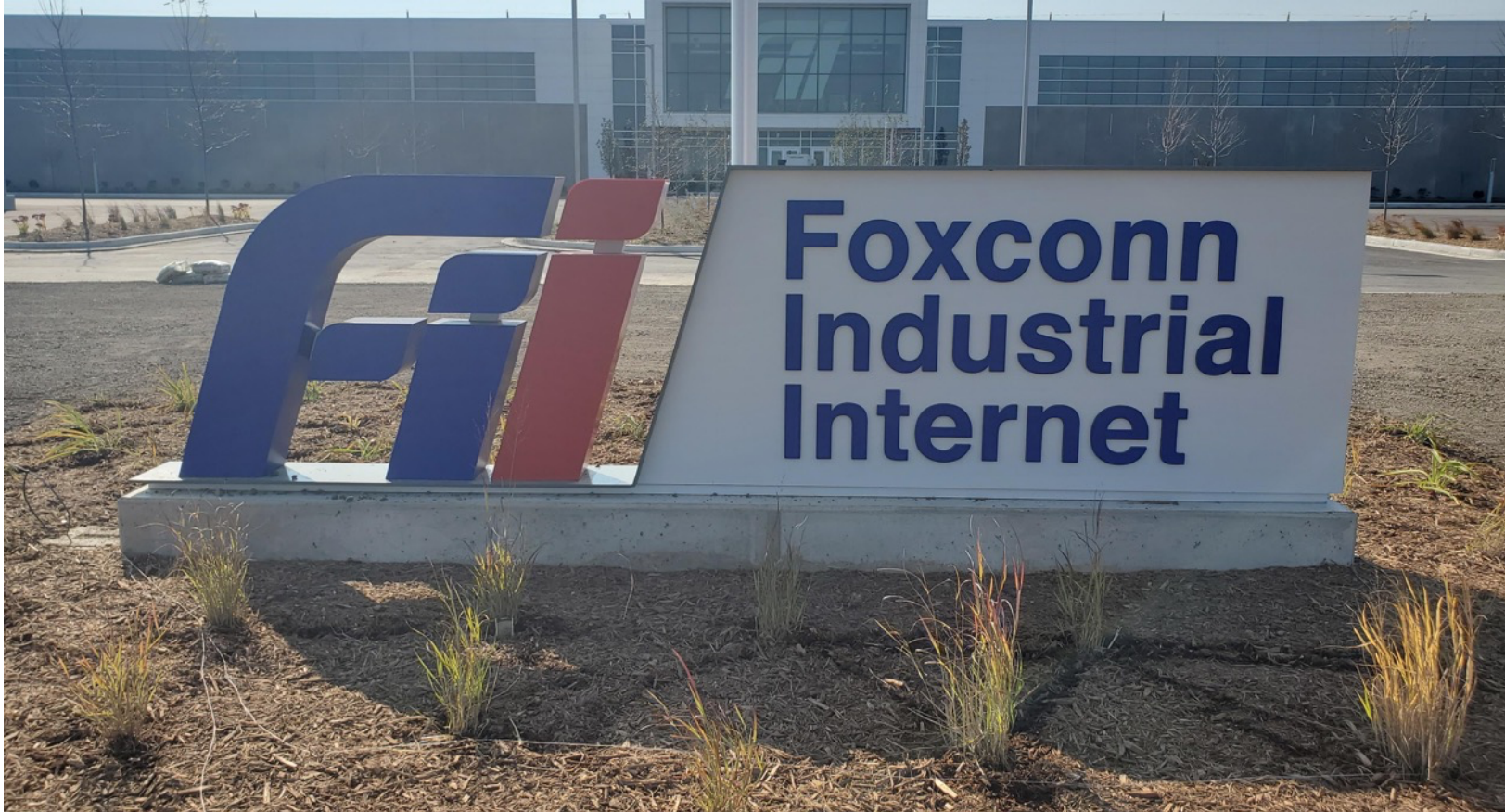
Installation of the 'Fii' monument sign and flag poles in the north parking lot
