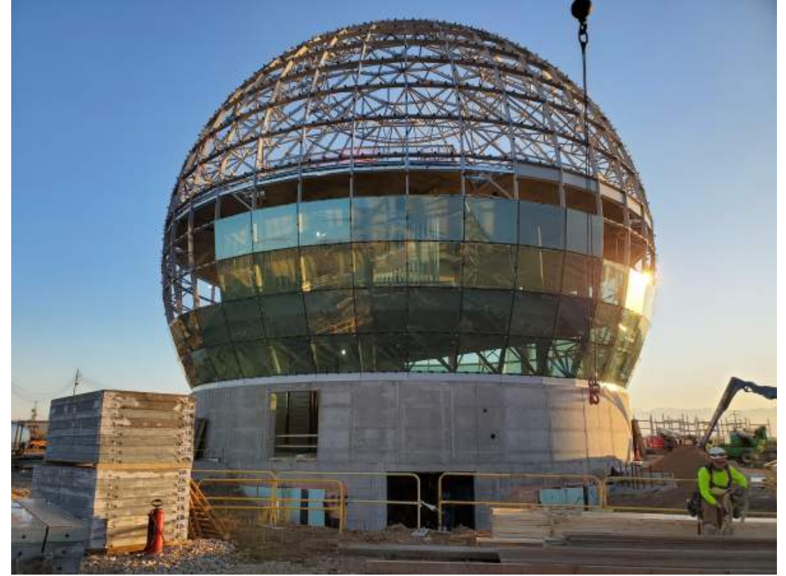
Begin glass installation on globe structure
