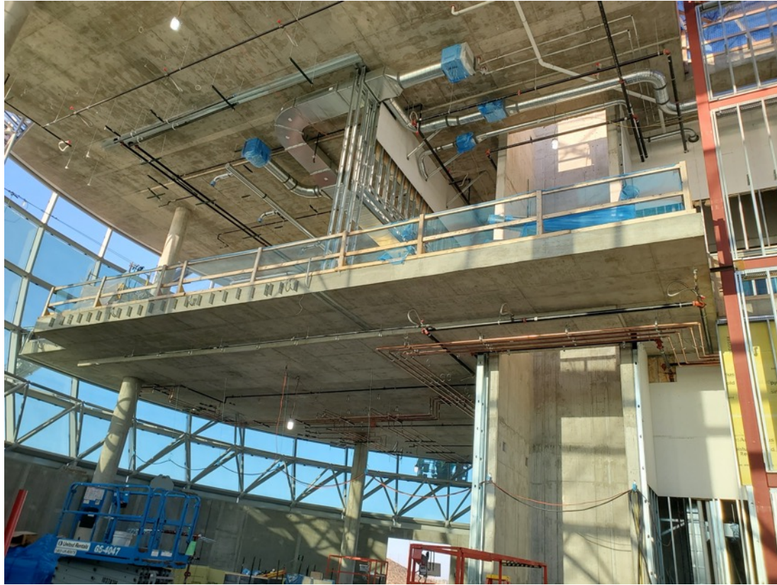
Overhead rough-in on 1 st & 2 nd floor
