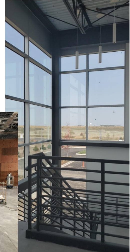
Complete lighting and painting in the stairwells
