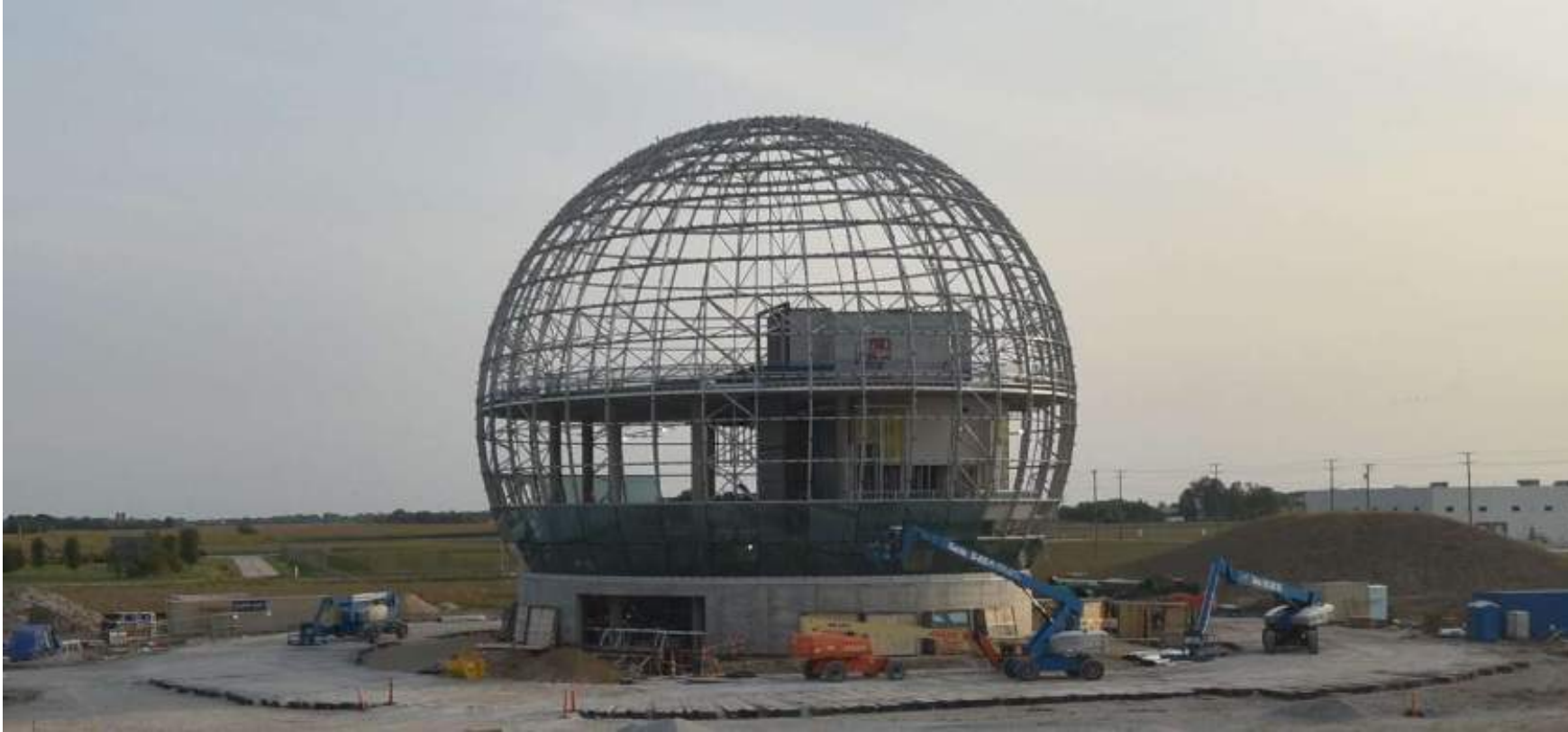
Data Center steel structure complete
